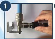
Slide sleeve to disconnect and exhaust air.
